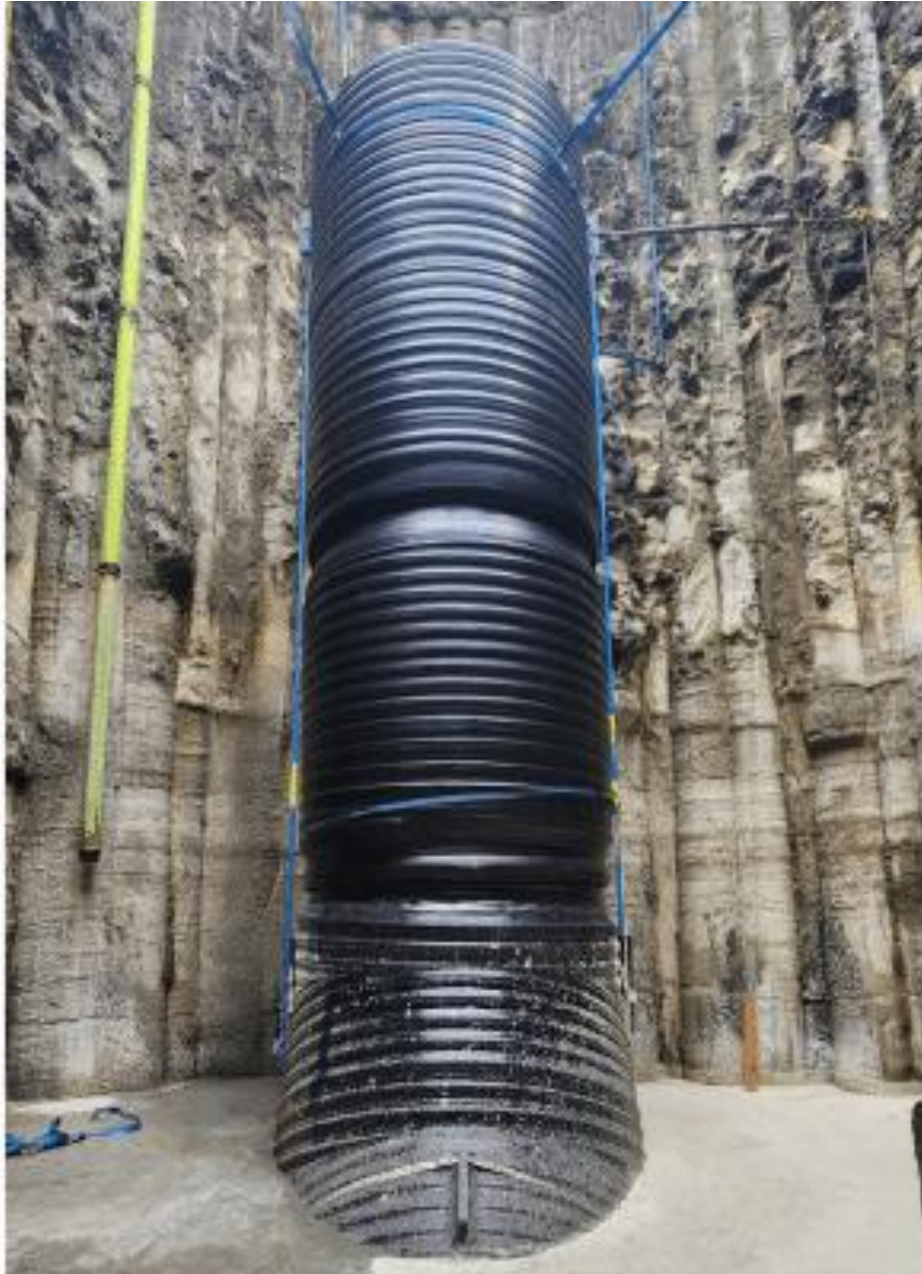
This photo shows the project once the riser has been installed
