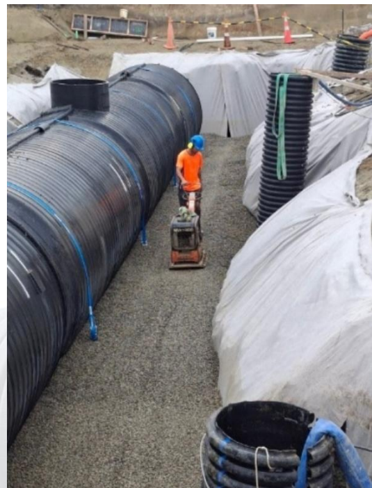
Compacting a partially backfilled tank
