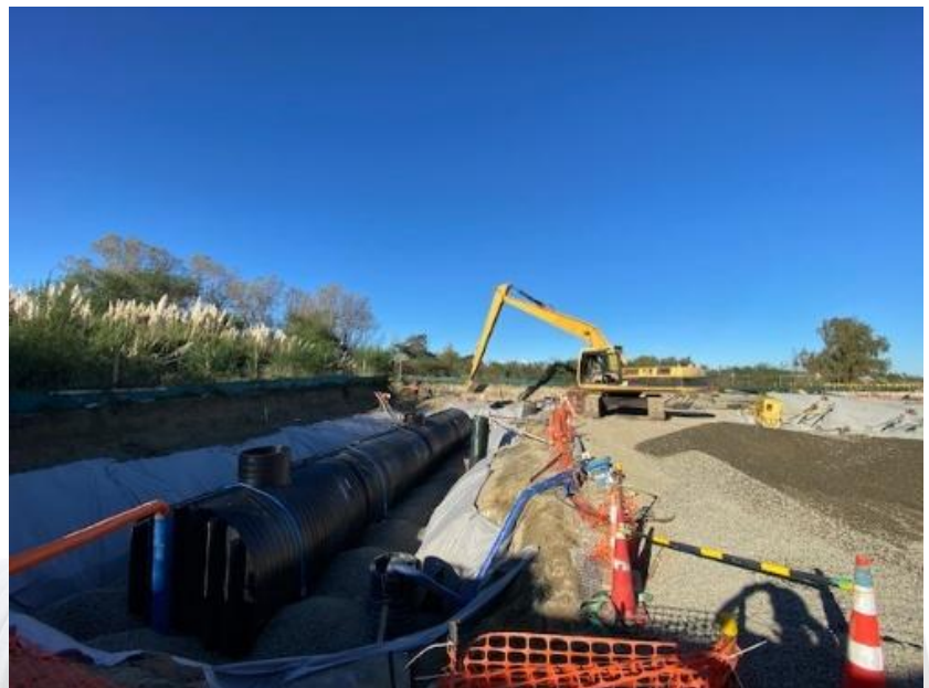
This 100m 3 buffer tank is in the Manawatu
