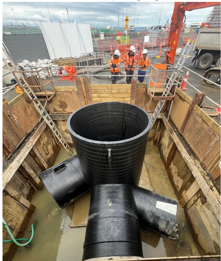
Fig 2. Airport manhole known as the 'turret'
