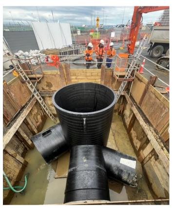
INFRAPIPE SOLID WALL is used for manholes efficiency.
